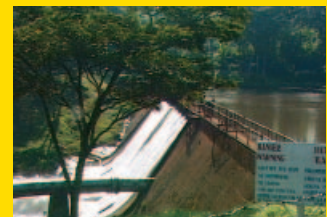
Hydro-electricity is generated from this reservoir on Unilever's tea estate in Kericho, Kenya. The estate also uses wood specially grown on the estate to fuel the boiler.
